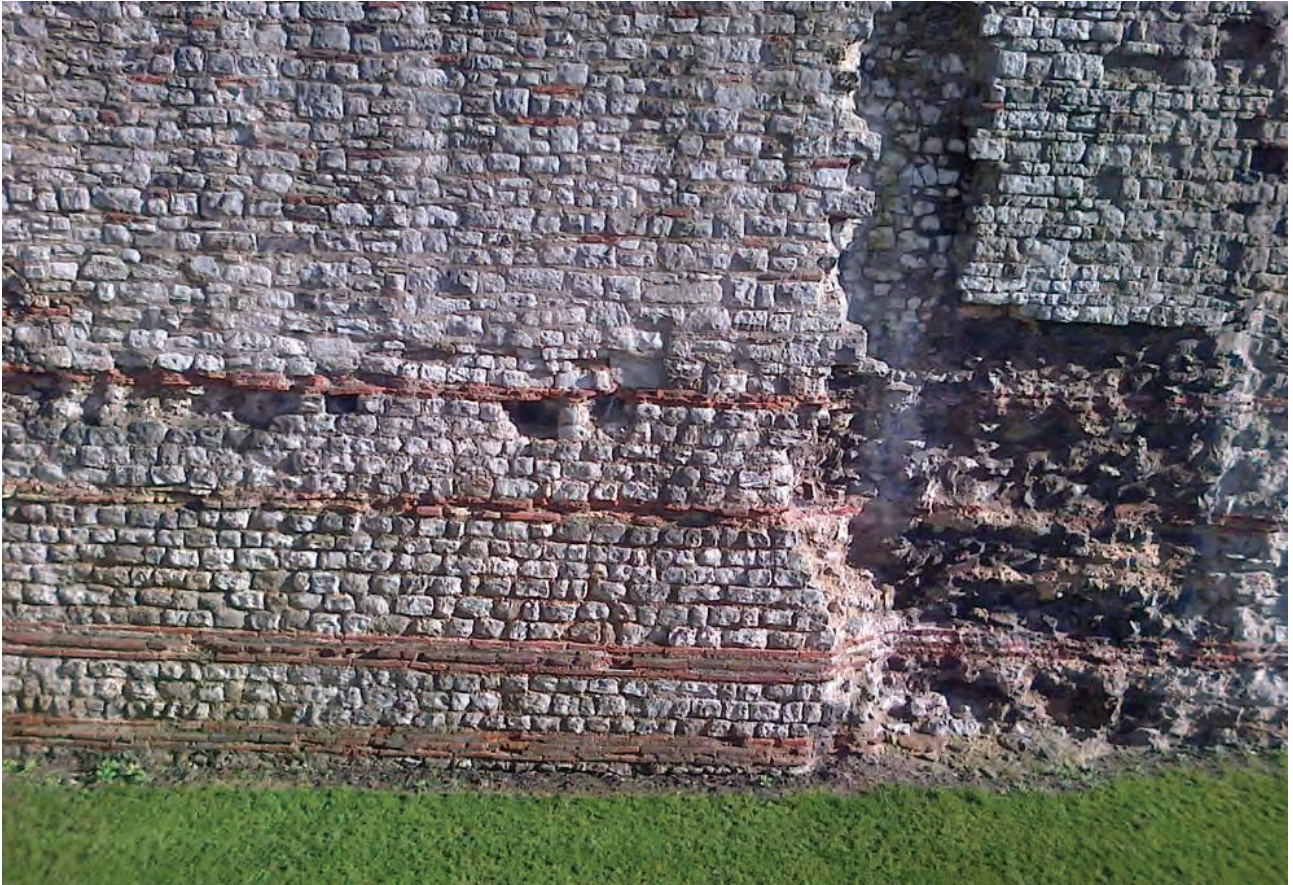
Finely worked upper Medway Valley Kentish ragstone blocks in the land wall of Roman London (this location near Tower Hill), late 1 st century AD. Hall and Merrifield (1986, 28) said over one million squared and dressed ragstone blocks, from the five quarries identified for the first time in this research, would have been used for the inner and outer facing alone. Simon Elliott.
