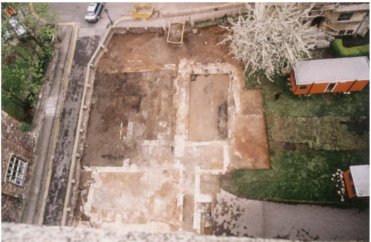
Fig. 5. View of the west end early in the excavation, seen from the cathedral south-west tower © Bristol Culture
